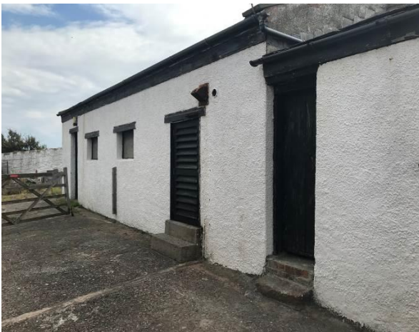
Fog Cottage east elevation, generator room to RH side
